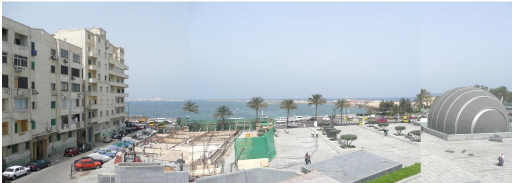
Figure 5: Panoramic view of the new building under construction.
